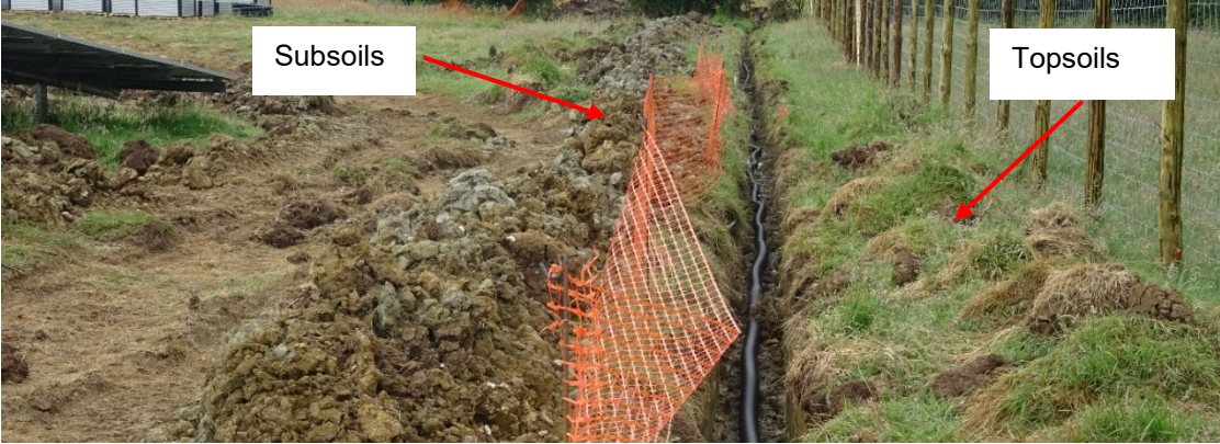
Insert 42: Subsoils Dug out of the Trench
